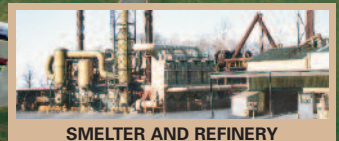
SMELTER AND REFINERY
